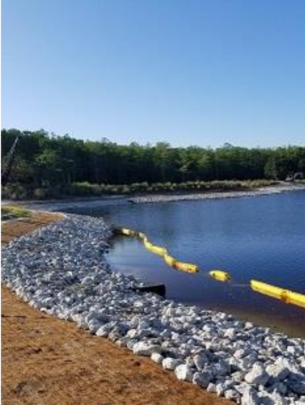
5/3/23 – Lake #64 – continued placing fill, geo fabric.
