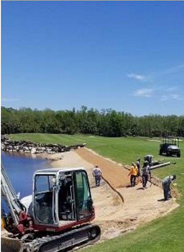
5/1/23 – Lake # 59, Hole # 7 Option # 3. Began placing fill dirt and coconut blanket
