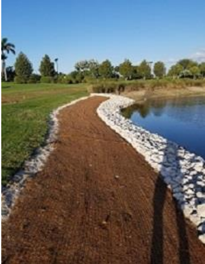
Lake #40, Hole # 1 - Completed placing fill dirt, geo fabric, riprap, and coconut blanket
