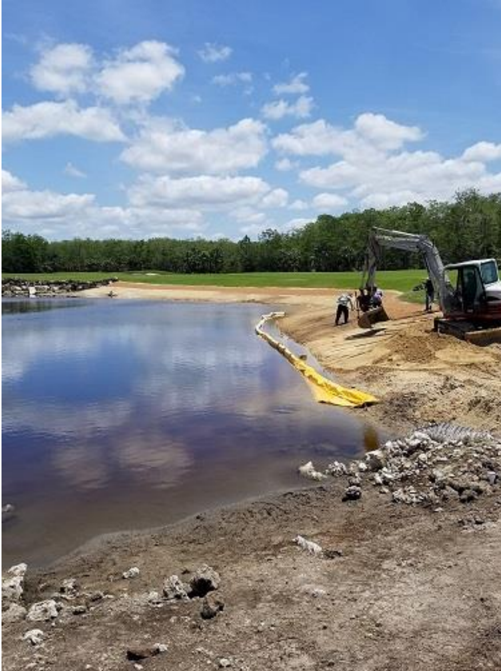
5/3/23 – Lake #59, Hole # 7 - Completed fill and coconut blanket installations
